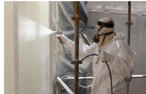
Application of high performance elastomeric urethane
