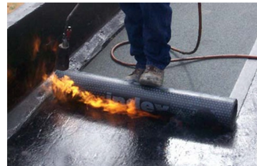
Torch applied waterproofing membrane
